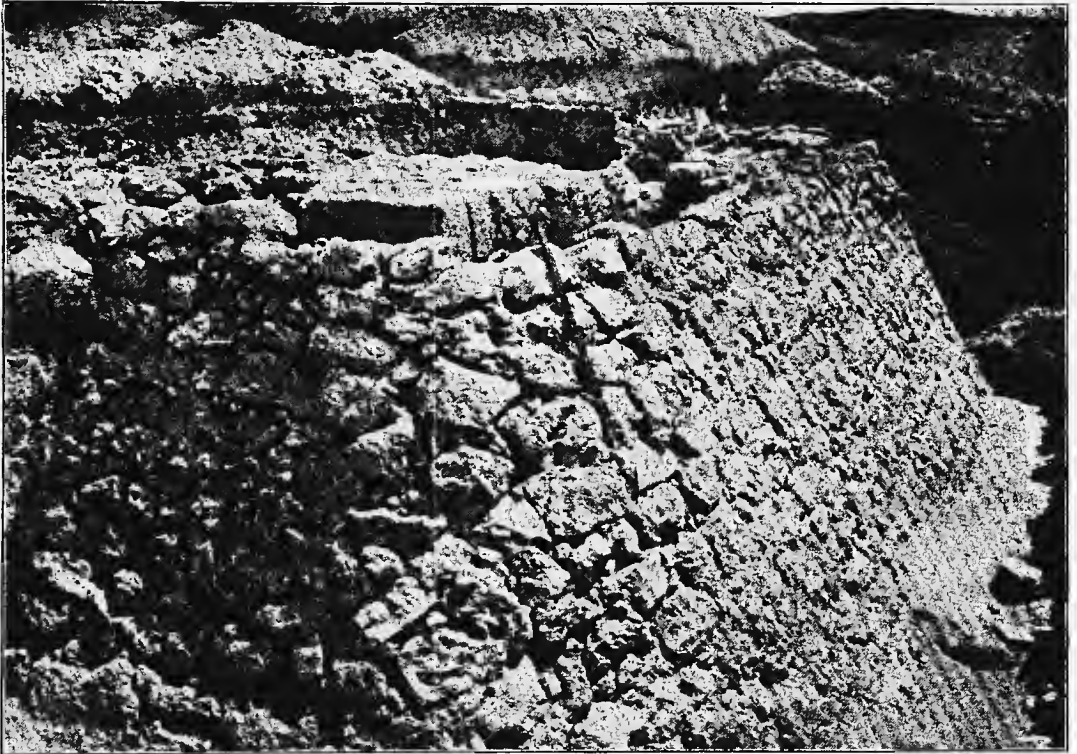
FIG. 128.—TOWER WITH BASTION
